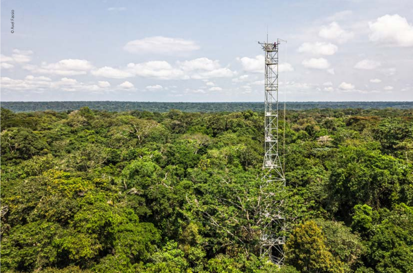
▼ The Congoflux tower in the Yangambi Biosphere Reserve (DRC) collects data to gain a better understanding of how carbon is sequestered.
